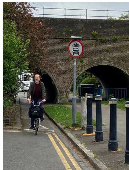
Cycle and Pedestrian access under railway bridge on Barry Avenue, Windsor
